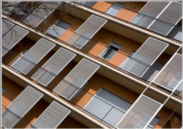
Housing. Granollers. Architect: Josep Sánchez Ferrer.
