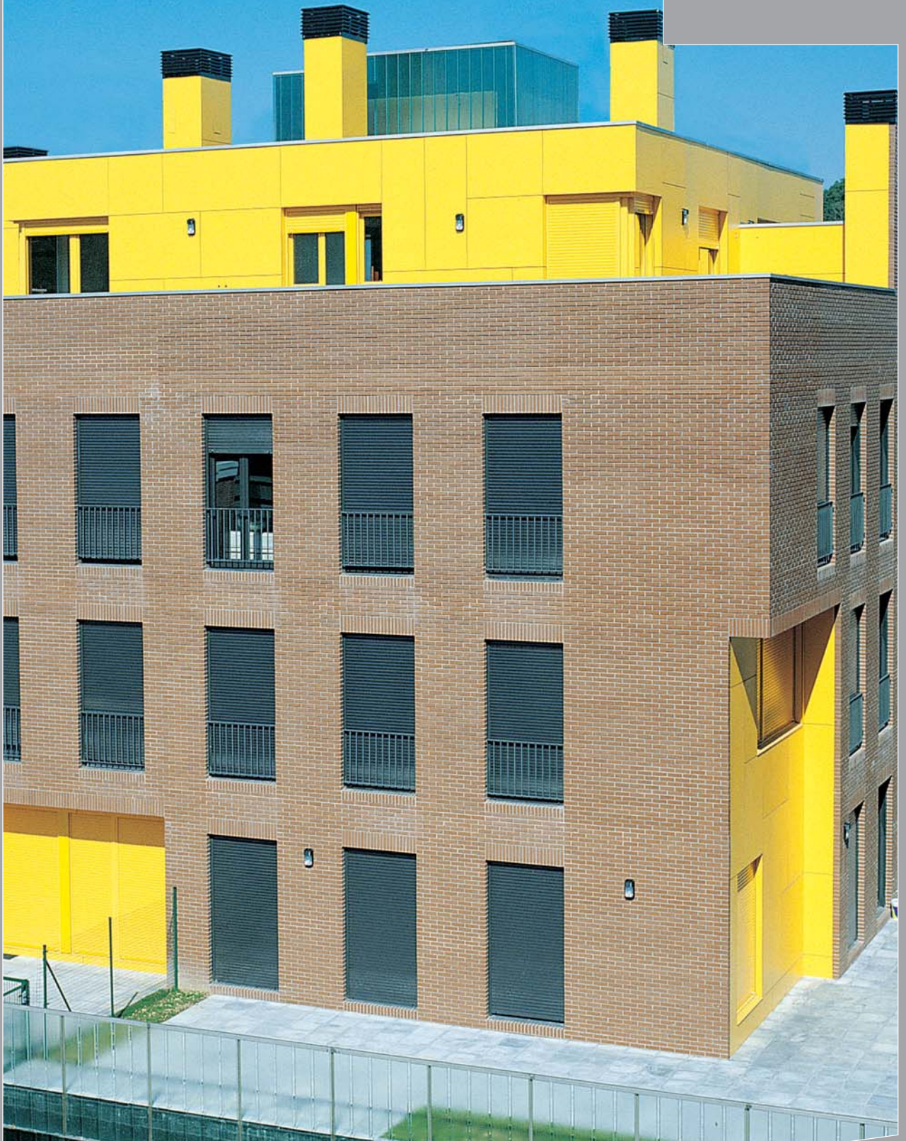
0.4 Private housing Sopelana, Spain Architect: Iñigo Piñera
