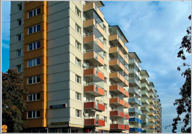
Housing. Kopparstaven. Sweden. Architecture: WSP Arkitektur.
